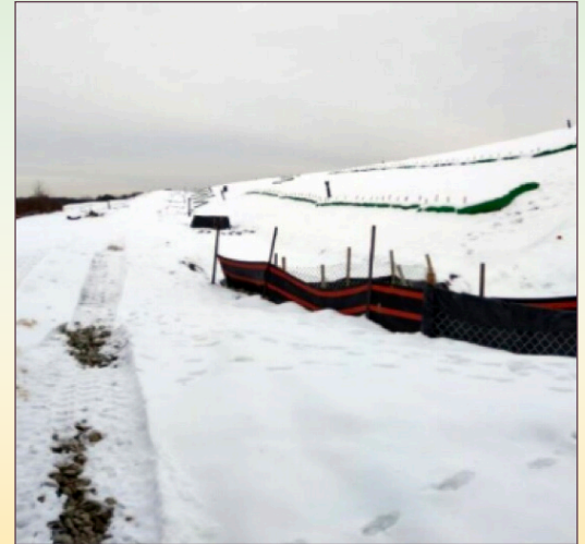
January snows on the working face at the Gude Remediation Project
