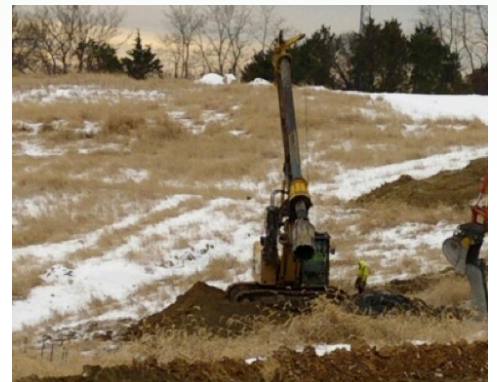
A large drill rig makes the holes to install LFG extraction wells in Phase IV
