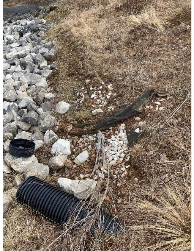
Exposed liner on top of Cell 3 Hypalon Ditch #3 (9)
