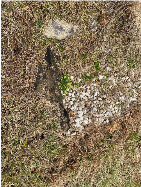
Multiple areas with erosion and exposed liners on Cell 7 Southeast slope (1)
