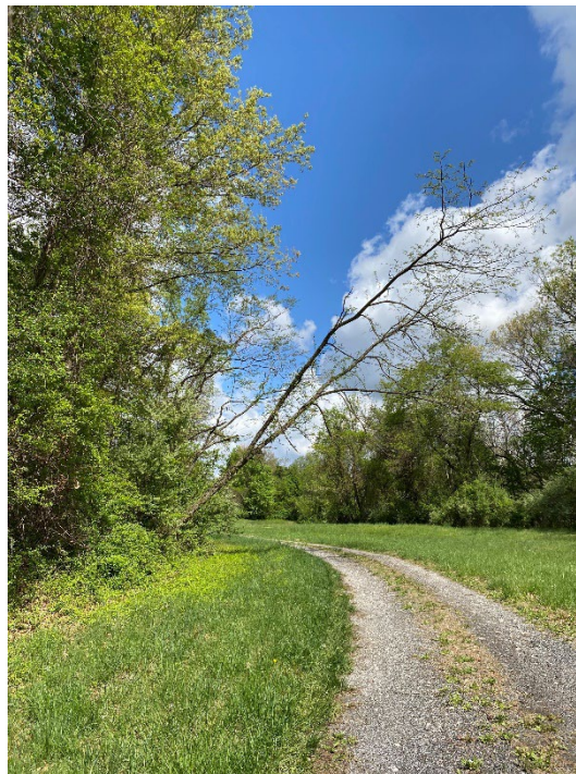
Falling tree over cell access road, near Basin D
