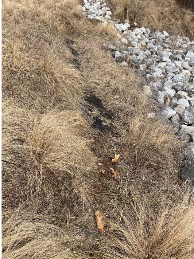
Exposed liner on top of Cell 3 Hypalon Ditch #3 (9)
