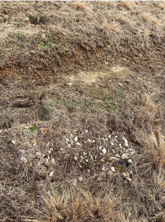
Erosion and exposure of liners on Cell 4 South-facing upper slope (4)
