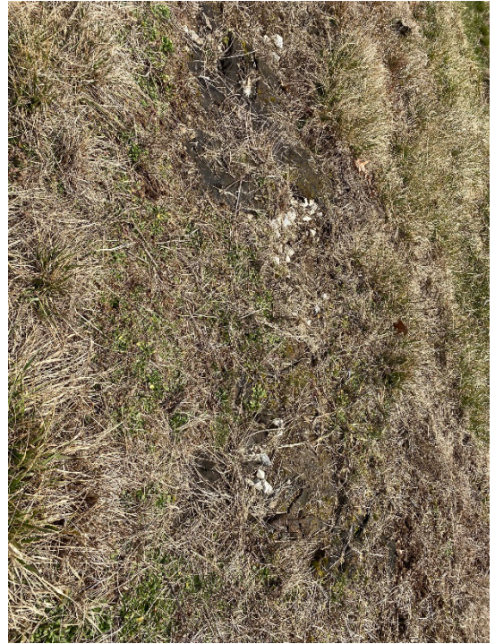
Areas with exposed liner on Cell 1 South-facing upper terrace (2)
