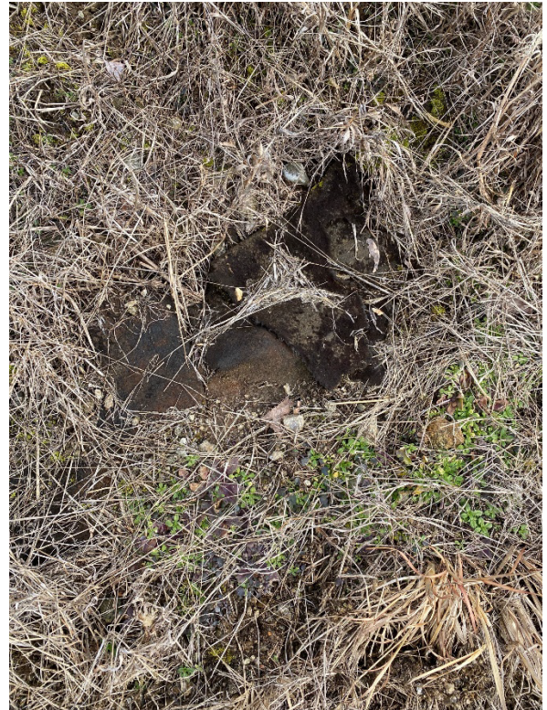
Erosion and exposure of liners on Cell 4 South-facing upper slope (4)
