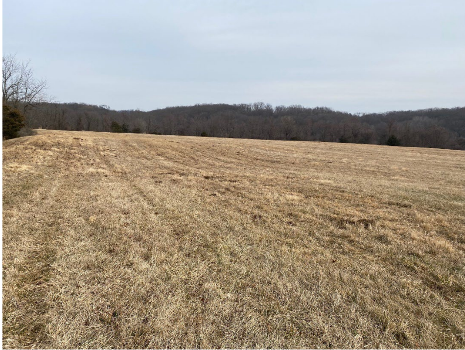
Settling on Cell 3 top cap (8)
