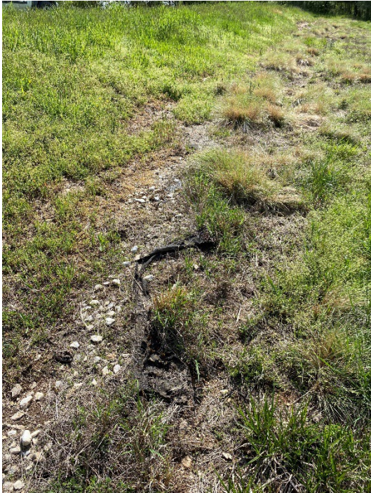
Erosion and exposed liners on Southern-facing slope
