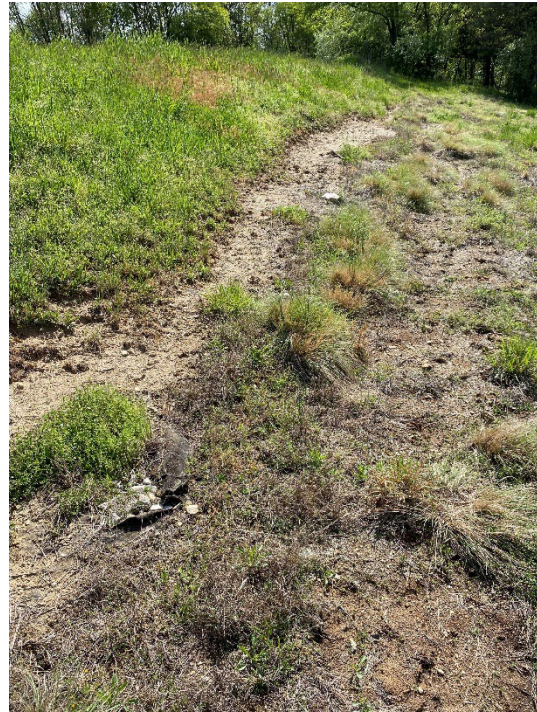
Erosion and exposed liners on Southern-facing slope
