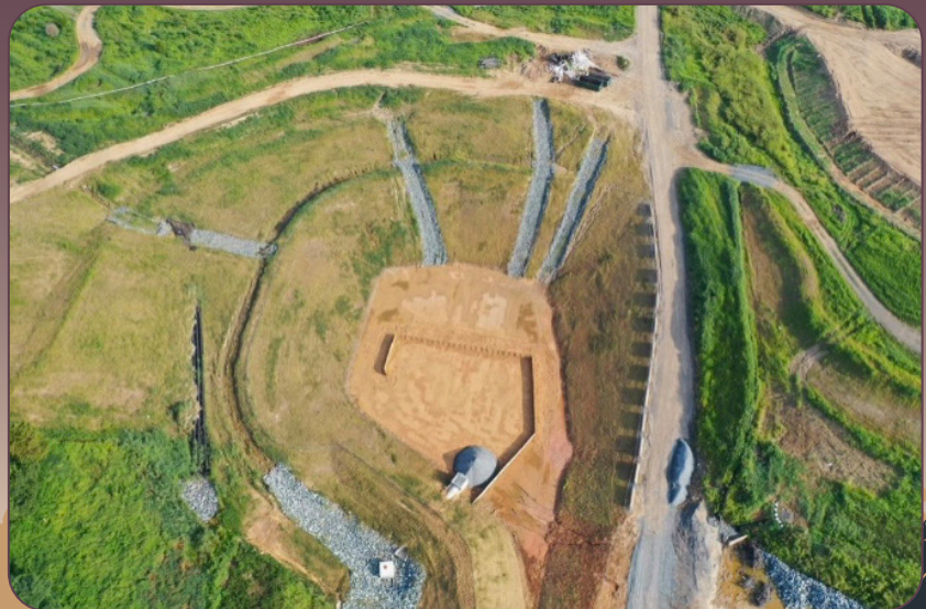
Aerial photo of Sediment Basin No. 1
