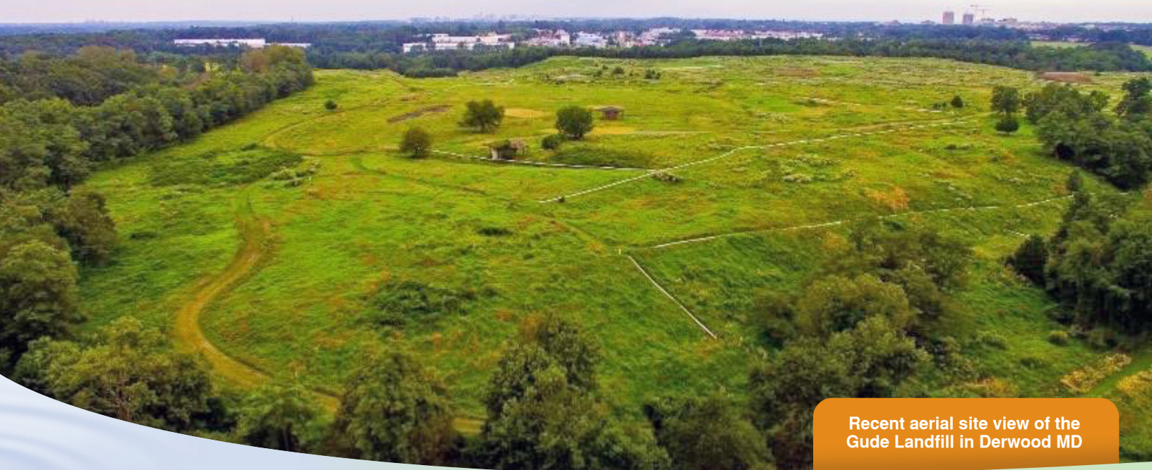
Example waystation on a landfill walking trail
