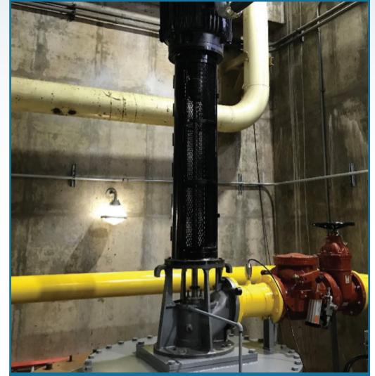
Pumps and piping installation complete
