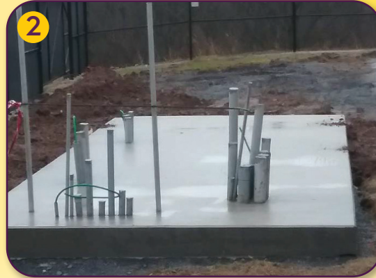
BESS Pad with conduit stub-ups after concrete pour. (01.03.2020)
