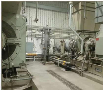
Turbines at the landfill gas-to-energy facility.
