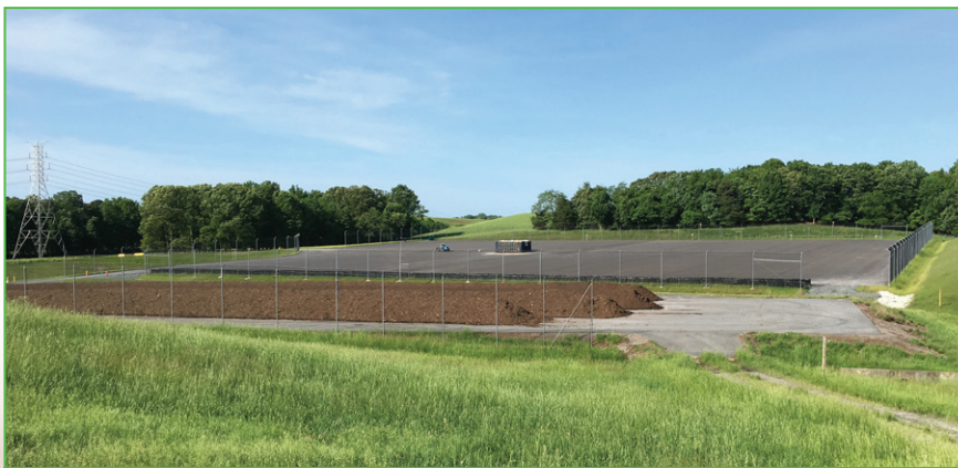
Completed compost pad.
