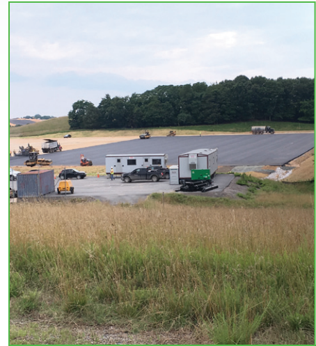
Compost pad under construction.
