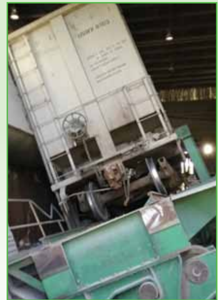
Railcar of waste about to be turned and dumped onto tipping floor
