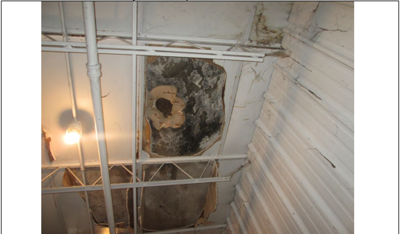
Photo No. 28: View of multi-layered ceiling material observed in the Loading Dock area of the Garage which was determined not to contain asbestos via PLM analysis of bulk samples.
