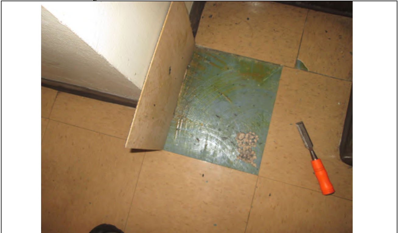
Photo No. 14: View of 12x12 tan VFT with associated yellow mastic overlying blue/green floor coating in the Office area. These materials were determined not to contain asbestos via PLM analysis of bulk samples. However, residual black VFT mastic on concrete slab (visible below the blue/green floor coating) is asbestos-containing.
