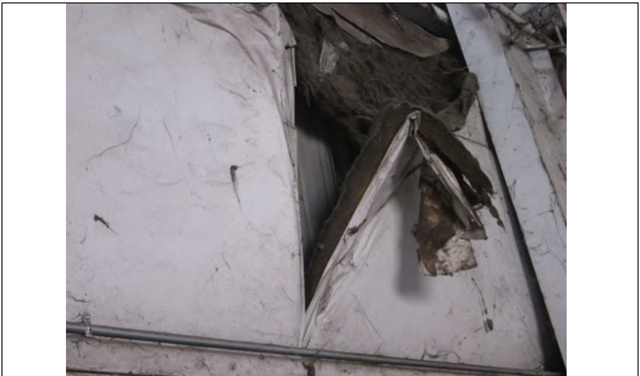
Photo No. 24: View of fiberglass insulation on corrugated metal Garage walls.
