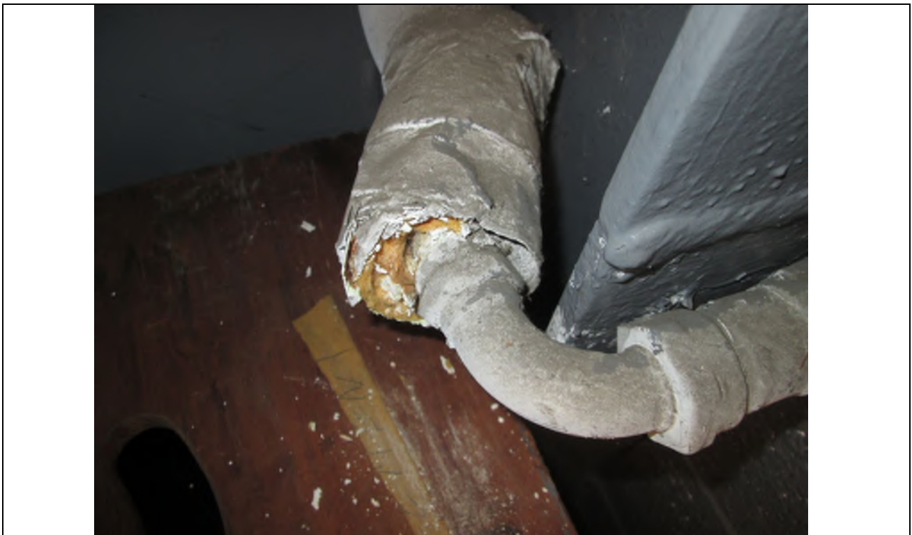
Photo No. 22: View of white end cap mastic/seam sealant on fiberglass pipe insulation found in the Garage area determined not to contain asbestos via PLM analysis of bulk samples.
