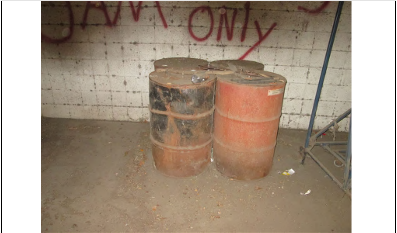
Photo No. 23: View of 55-gallon drums observed in the Garage area.
