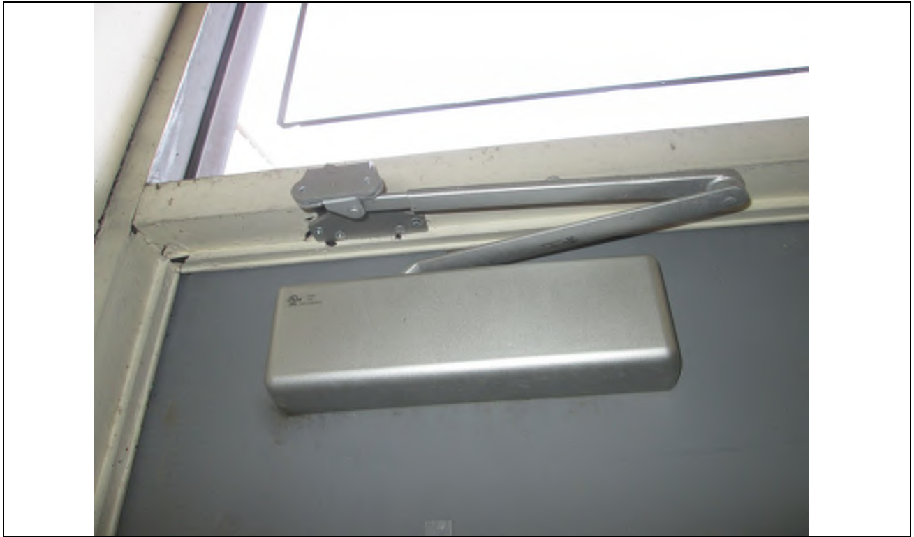
Photo No. 15: View of typical door closer observed in the building which is presumed to contain an oil reservoir.
