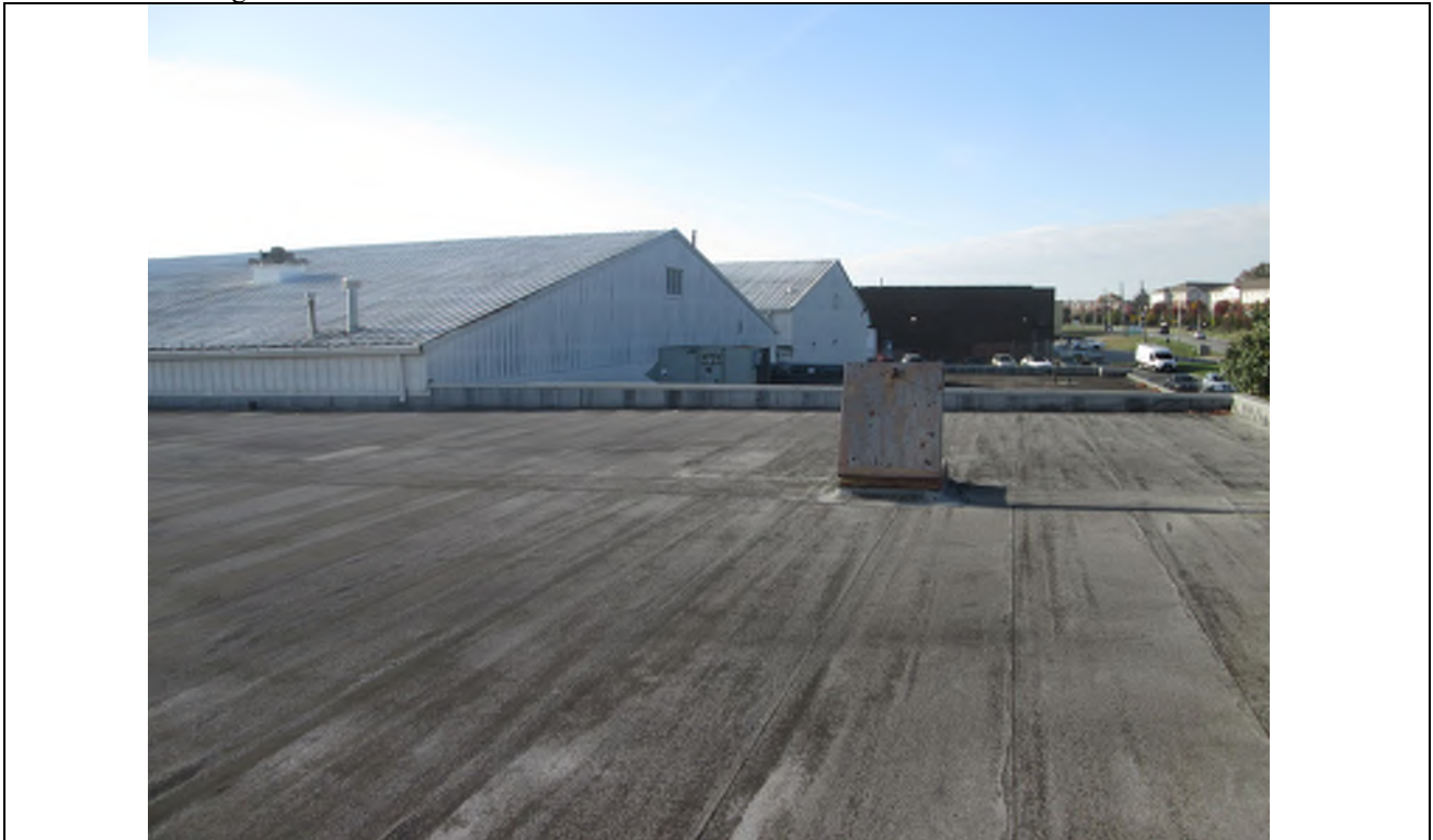
Photo No. 26: View of building roofs. The Warehouse roof and a portion of the Garage roof were accessible during the survey. Inaccessible roofing areas did appear to be consistent with accessible roofing components.
