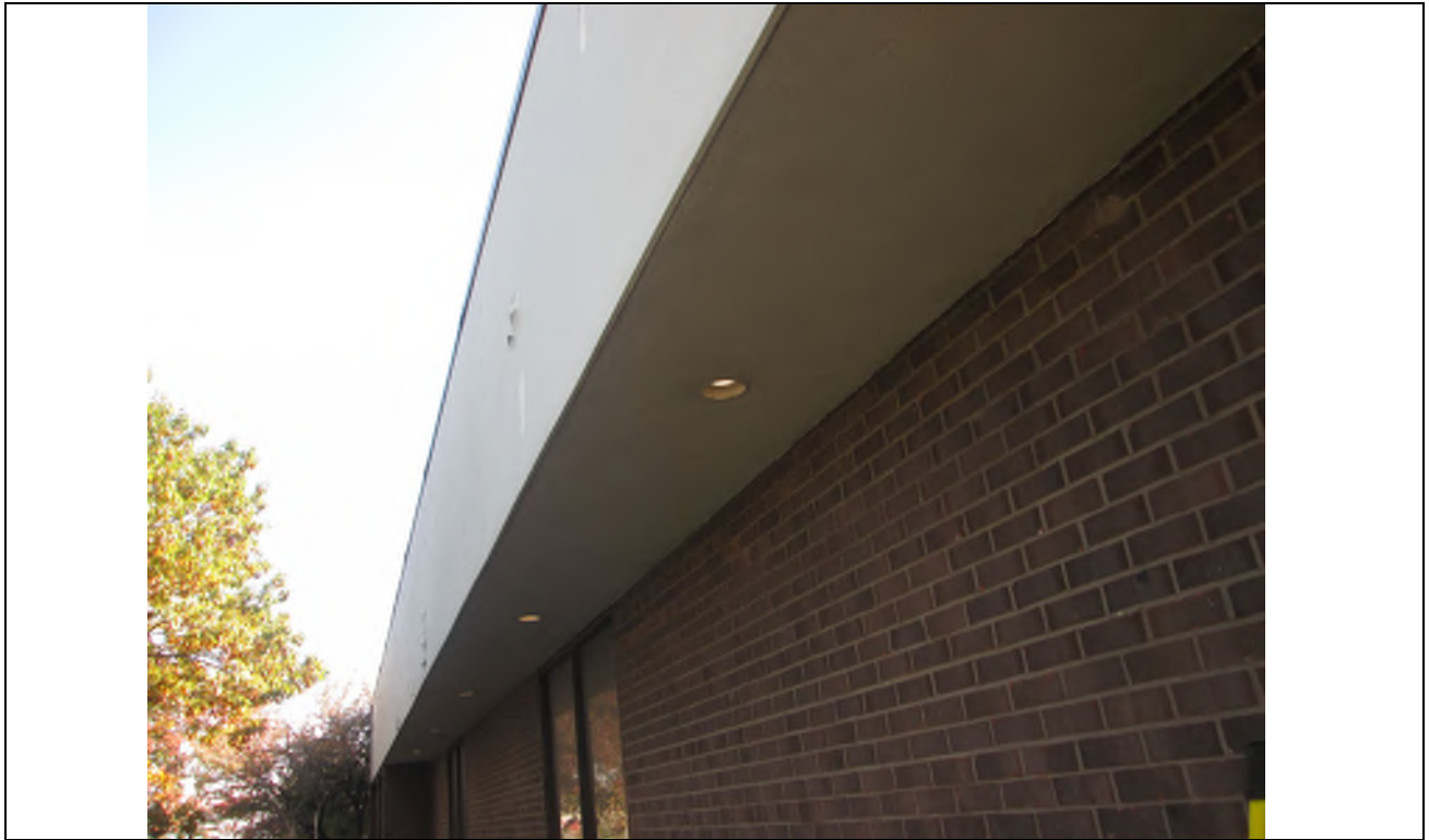
Photo No. 27: View of exterior fascia/soffit on Office area. The cementitious soffit material was determined not to contain asbestos via PLM analysis of bulk samples.
