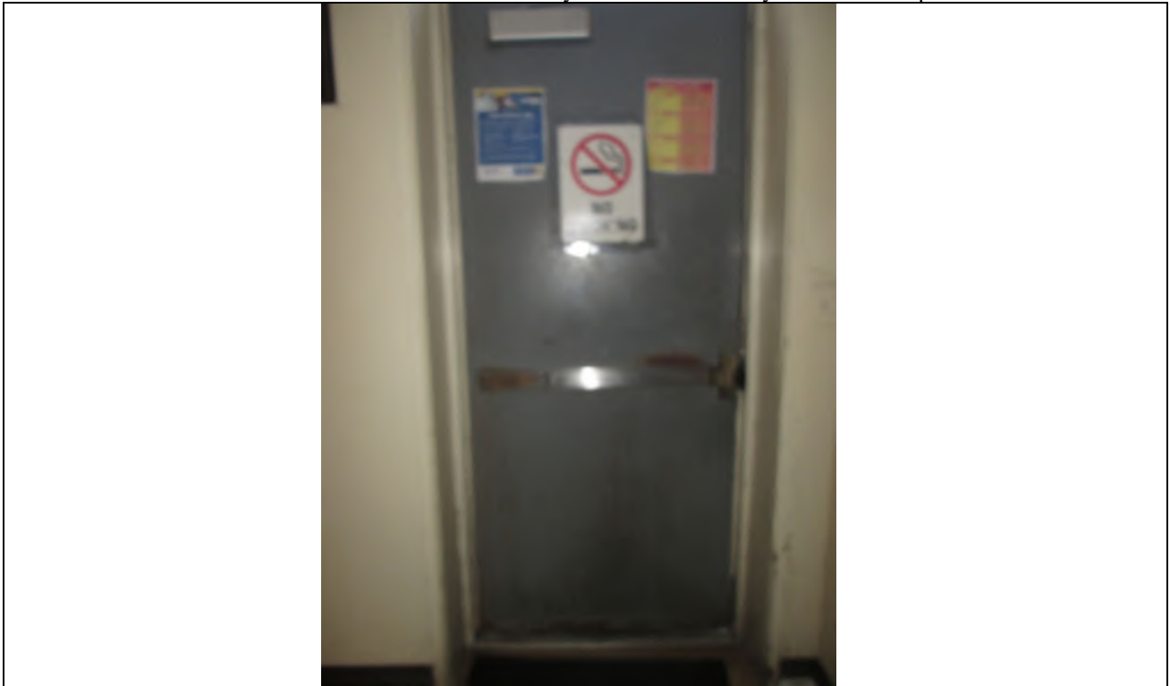
Photo No. 6: View of typical metal fire door observed in the surveyed areas presumed to be asbestos containing.
