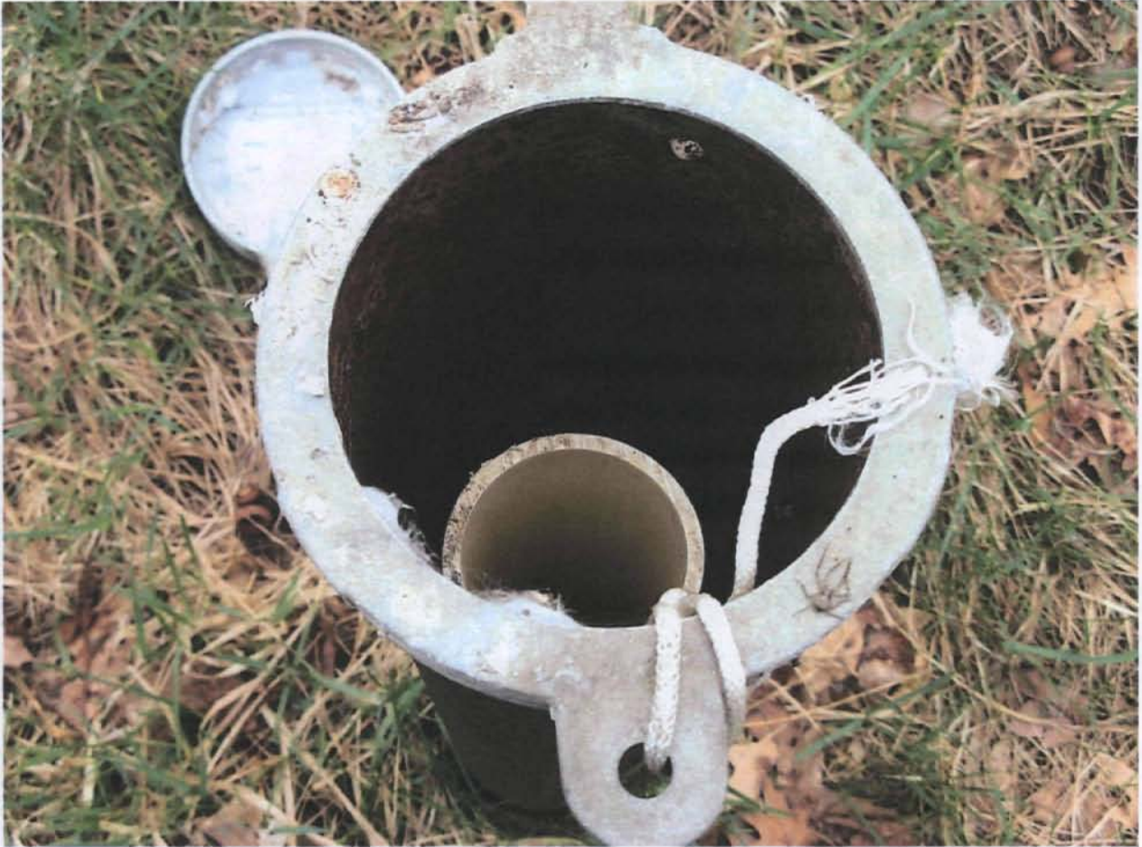
Figure 13. Unidentified well without lock.
