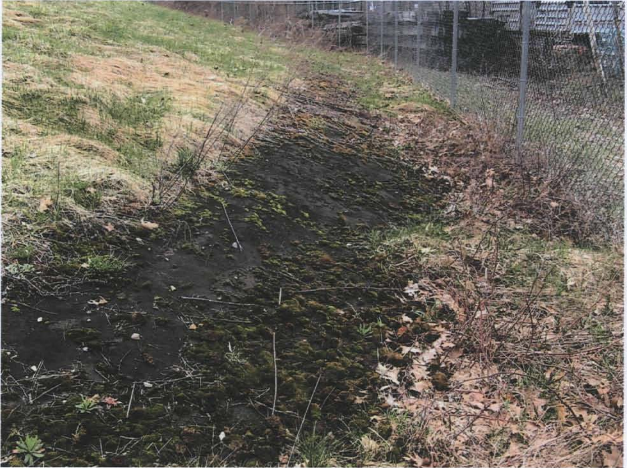
Figure 18. View of geotextile exposed
