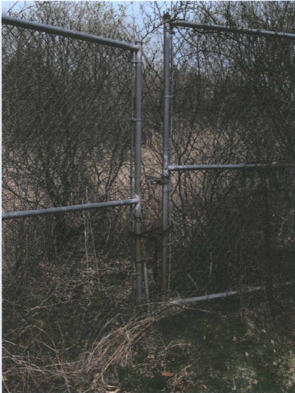
Figure 23. Unlocked pedestrian gate at western side of the fence.
