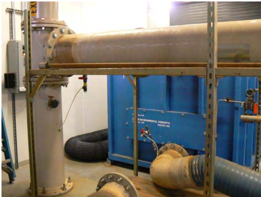
Photo 6: VOCs are removed from the stripper air by carbon filters (shown in blue). The carbon in the carbon filters is eventually disposed of in a hazardous waste landfill.
