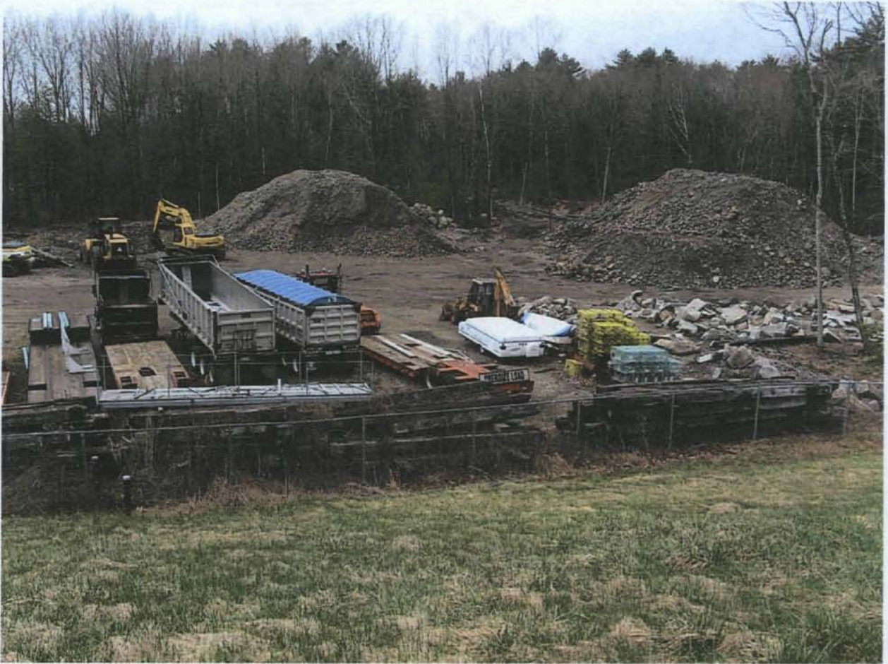
Figure 16. View of construction equipment depot along the southwestern section of the fence (looking south from the top of the landfill)
