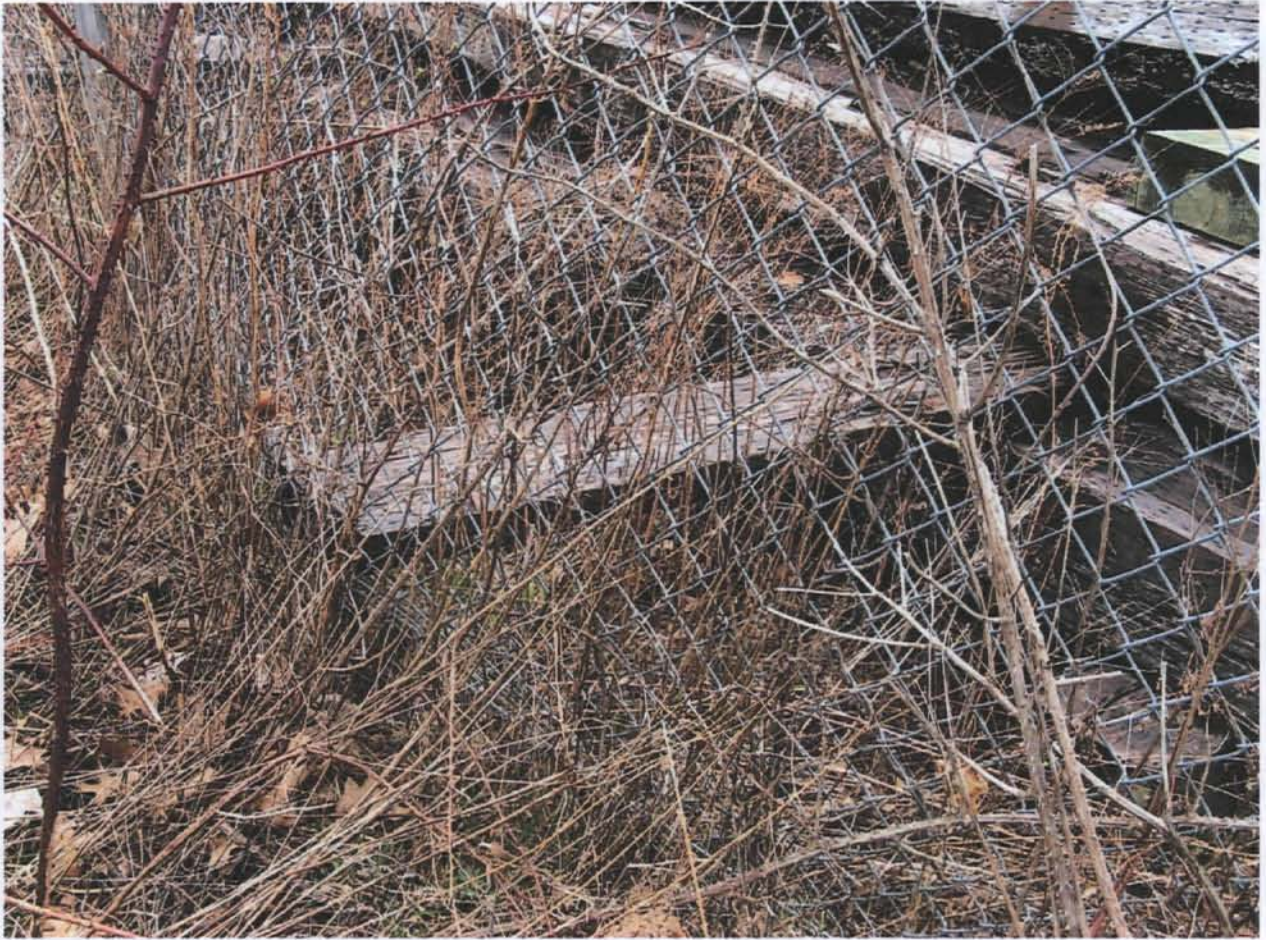
Figure 17. View of wooden post protruding into the fence
