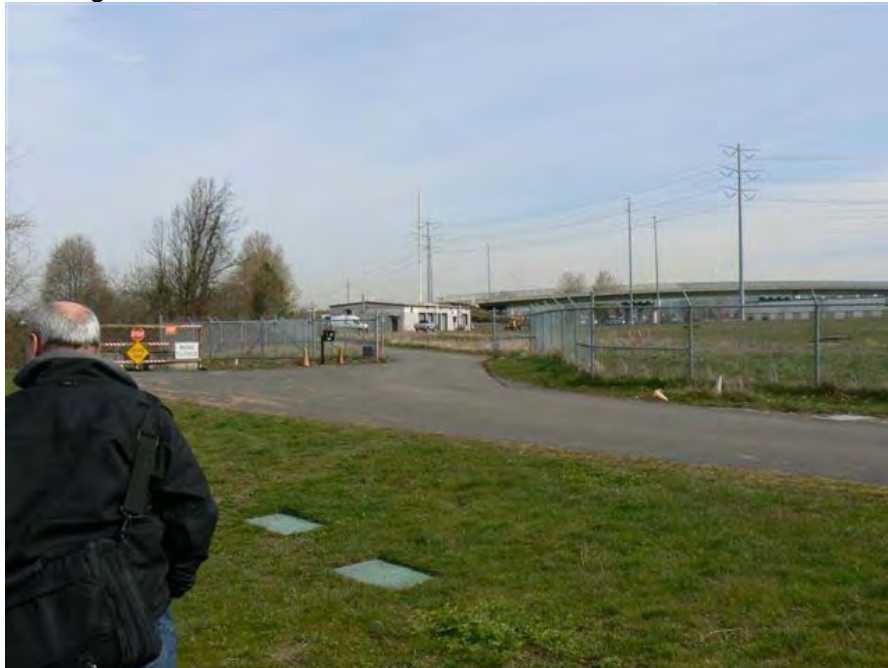
Photo 2: Immediately outside of the entrance. The gate was opened just prior to taking this photo to provide a better view of the road and the water treatment building. Sector 1 is behind the fence.
