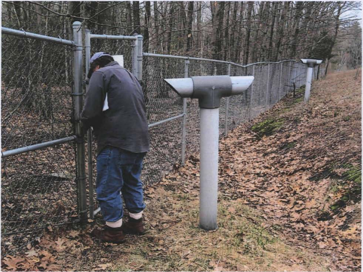
Figure 14. View of pedestrian gate at the Southeastern corner of the fence, gas vent, and partial erosion of the drainage slope's toe.
