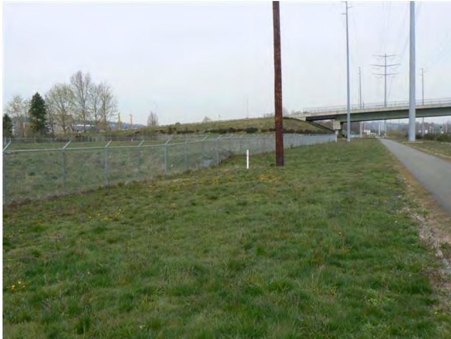
Photo 9: Interurban trail and the 196 th Street overpass. This view is towards the north. Sector 1 is on the left side of the fence line.
