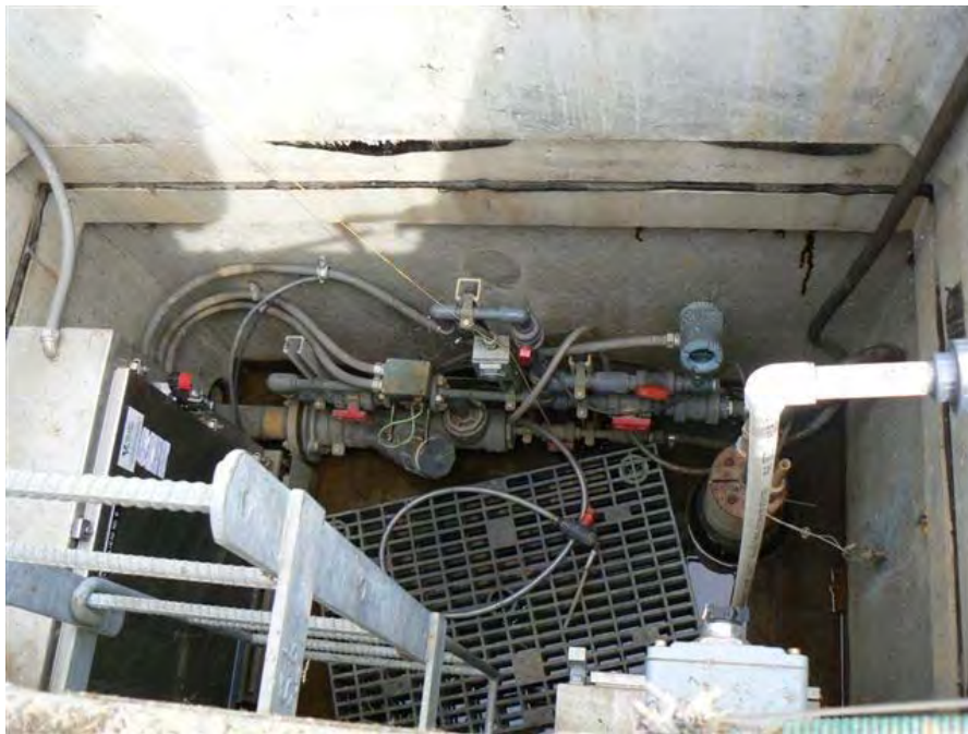
Photo 4: A view inside one of the extraction vaults.
