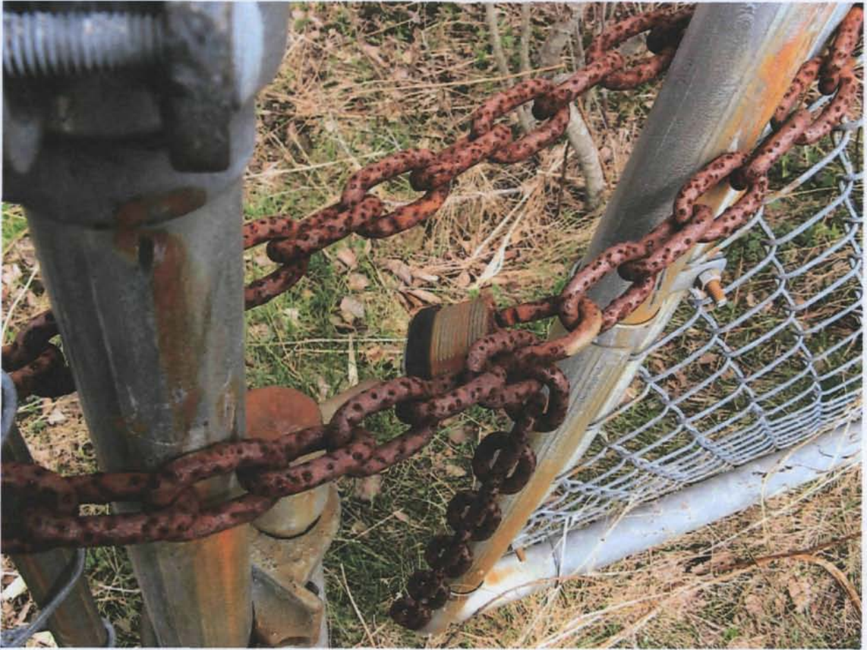
Figure 22. Unlocked pedestrian gate on the western side of the fence.
