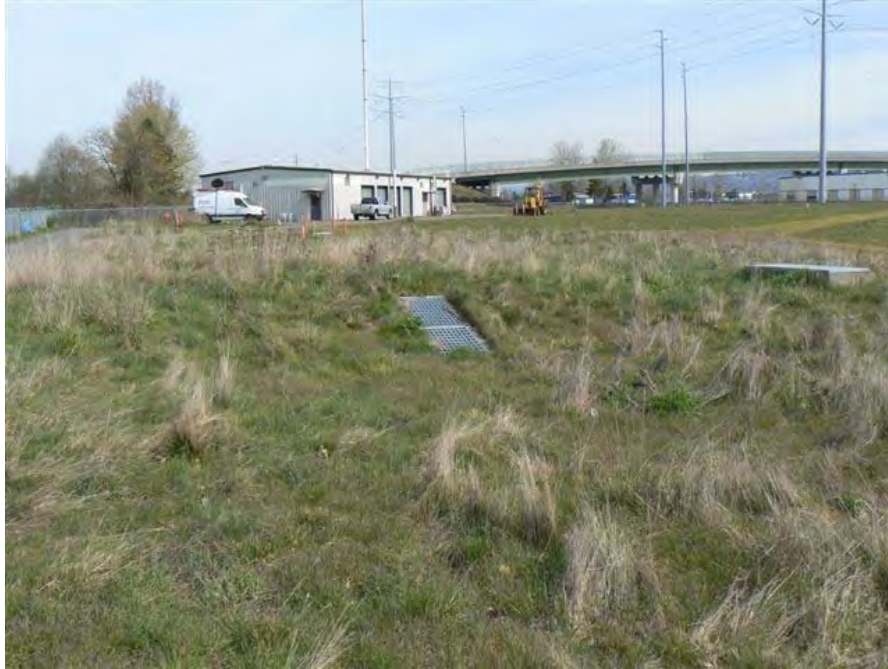
Photo 3: This photo was taken on top of the RCRA cap, looking north. One of the storm drains for the RCRA cap (center) is visible as is one of the extraction vaults (right center). The storm drain was kept clear of overgrowth. The water treatment building and the South 196 th Street bridge are both visible in the background.
