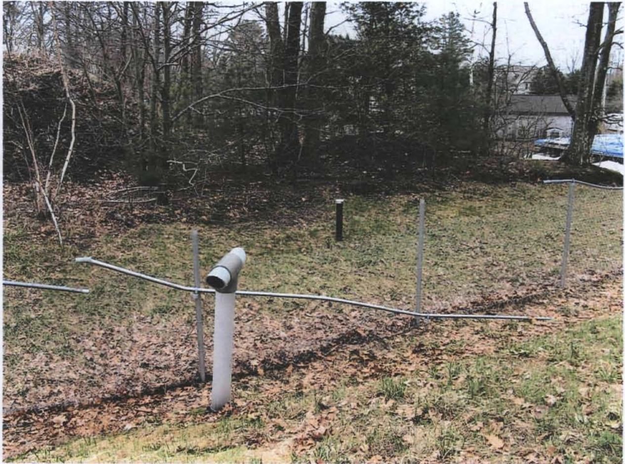
Figure 11. Damaged fence with well MW-4 in the background (Looking south)
