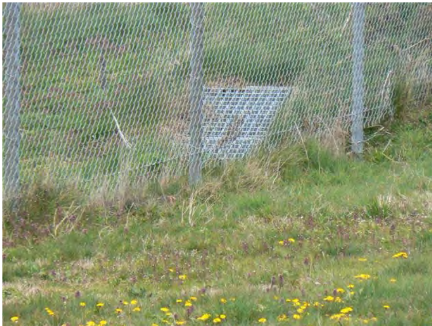
Photo 10: A storm drain in Sector 1 for the RCRA cap. The vegetation seen in this photo is in the foreground; the drain was clear of any overgrowth. The fence does not reach the ground at this location, but the reinforcement line near the bottom would still make access to the site rather difficult.
