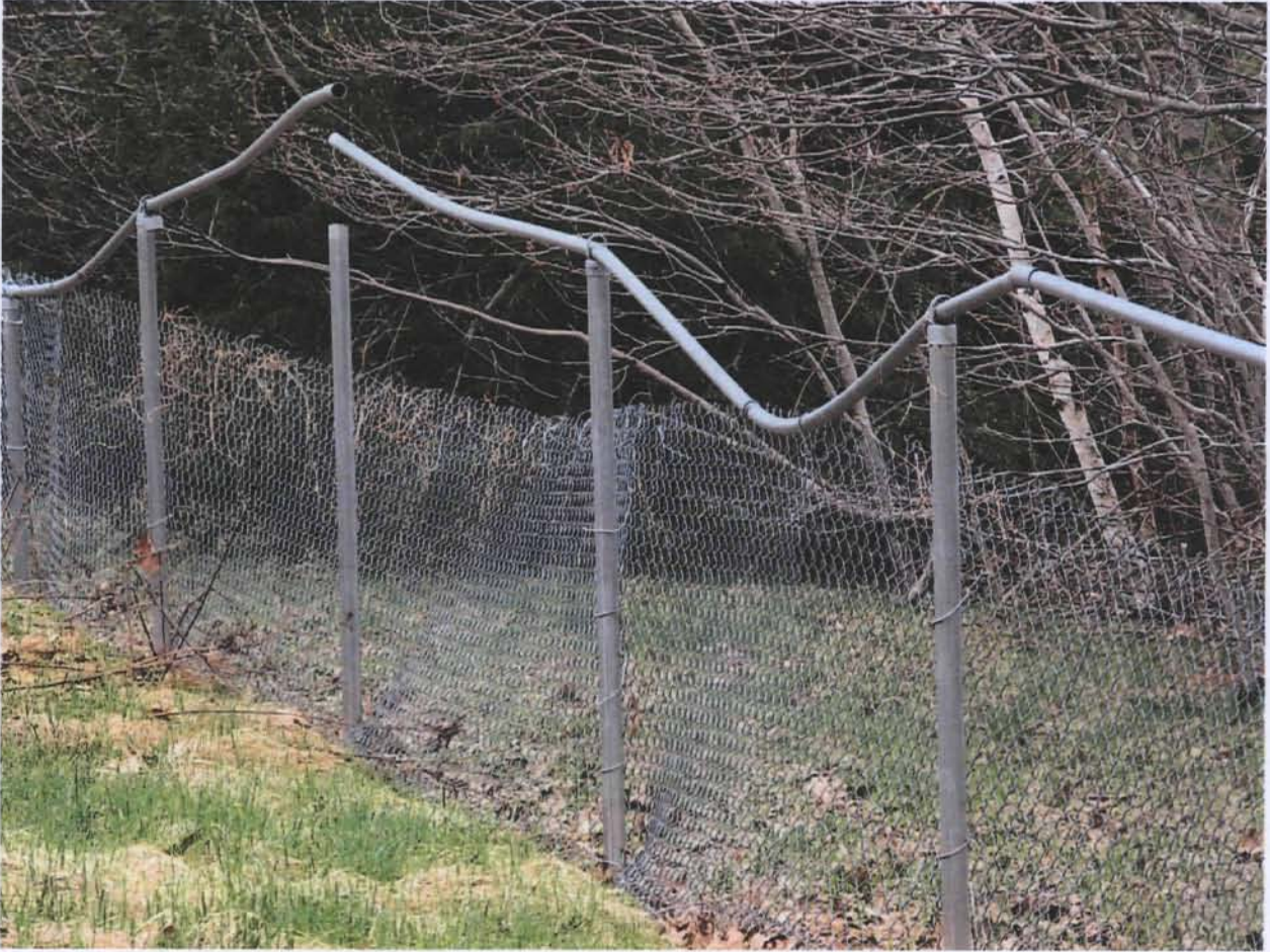
Figure 10. Snowstorm/ice damage to eastern section of the fence.
