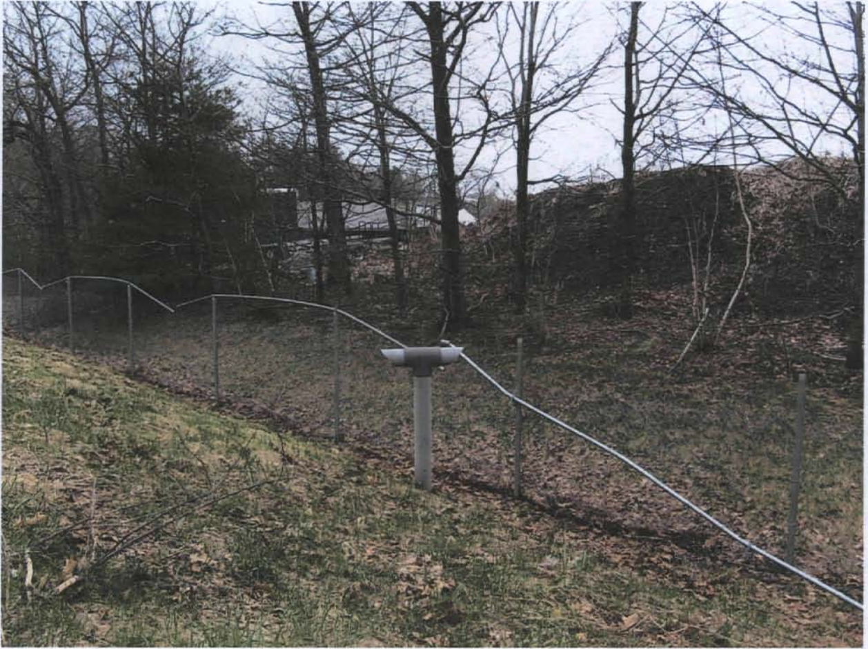
Figure 12. Damaged fence on the southern section (Looking south)
