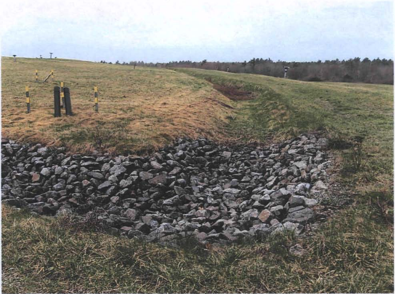
Figure 5. Rip-Rap on top of drainage swale. Looking west.
