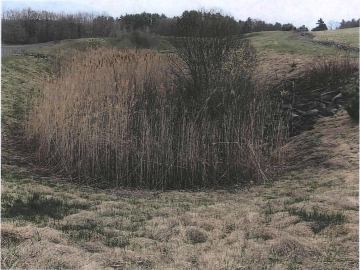
Figure 24. Overgrowth of vegetation on top of drainage swale.
