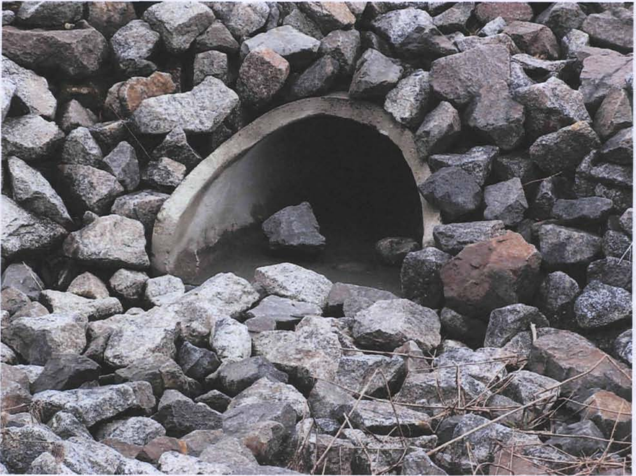
Figure 6. Drainage culvert showing partial obstruction from rip rap.
