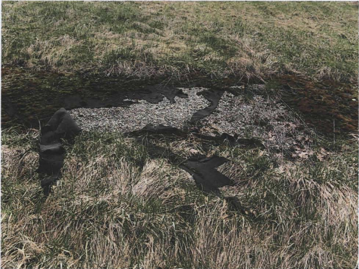
Figure 20. Section of the drainage slope (toe) showing rupture of the geotextile and exposure of the gravel underneath. Southwestern corner of the landfill.
