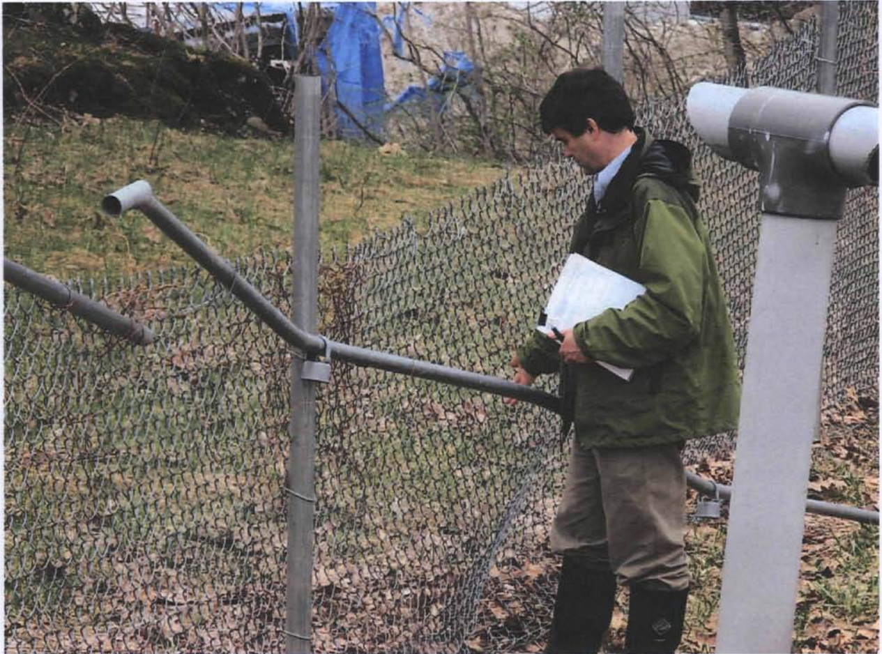
Figure 9. South-eastern section of fence showing snowstorm/ice damage
