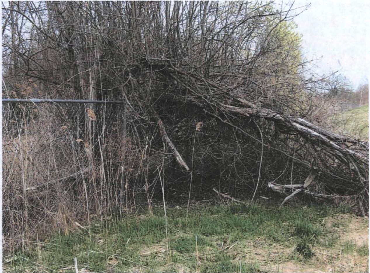
Figure 21. Fallen tree on top of a section of the western side of the fence. Looking north.
