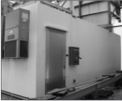
▲ A continuous emissions monitoring system will measure O 2 and SO 2 at the inlet of the Spray Dryer Absorber and CO, O 2 , SO 2 and NO x at the outlet of the electrostatic precipitator. This shelter will house the gas analyzers along with the data acquisition system.
