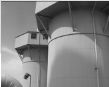
▲ Spray Dryer Absorbers #2 and #3 assembled and insulated.
