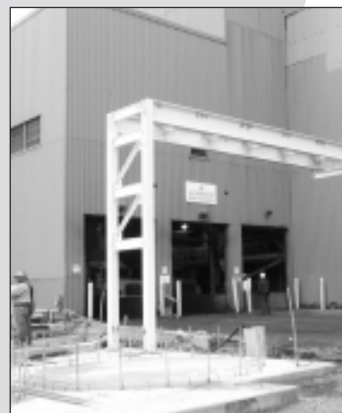
The pipe bridge will carry main process piping systems from the lime preparation building to the boiler building.
