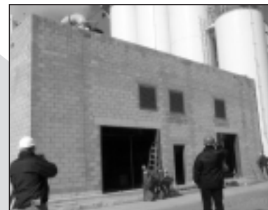
▲ Masonry walls have been constructed for the lime preparation building.
