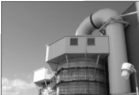
◀ Spray Dryer Absorber for unit #2 is fully assembled with penthouse and inlet duct.
