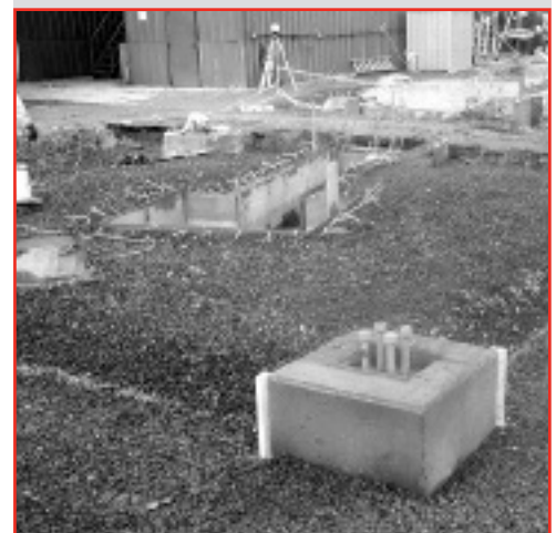
Nearly completed foundation for the acid gas scrubber.
