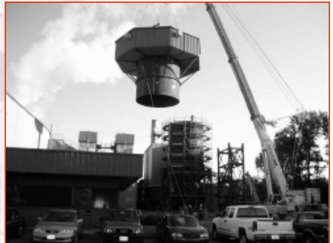
The scrubber continues its ascent.
