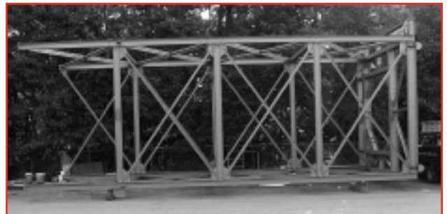
Large piece of support steel that will hold the new ductwork
